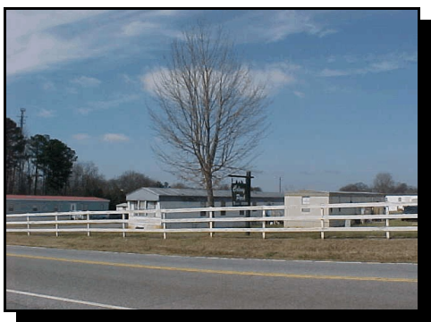
(6) Colony Park (MHP) north- west of site.
