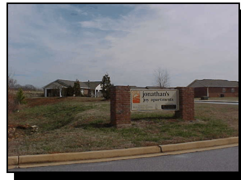
(4) Jonathan's Joy Apartments, west of site.
