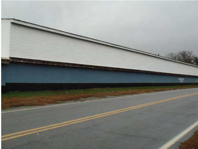
Adjacent Property. Mini storage warehouse across Lewis St
