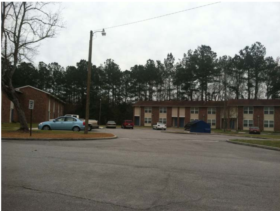
-Looking at northeast corner of site from within the property
