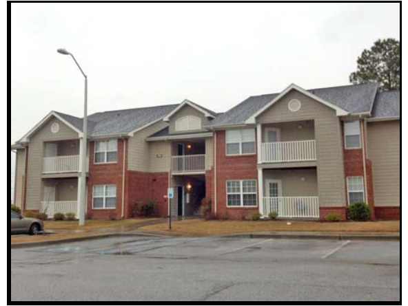
Typical existing building
