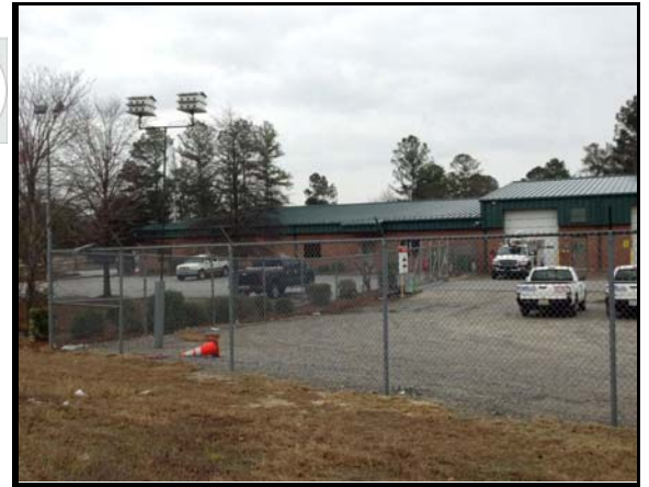
Northeast view from site
