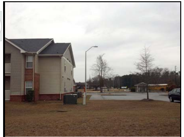
Northwest view from site
