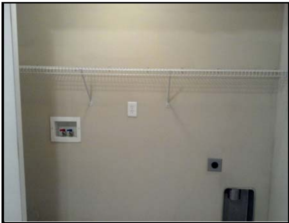
Typical accessible three-bedroom laundry area
