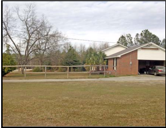
North view from site
