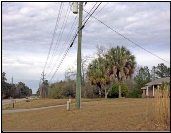
Power lines running north along east side of Columbia Road
