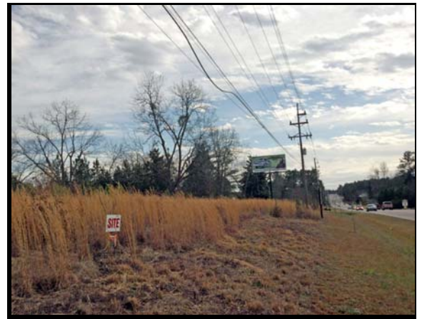
Power lines running south along east side of Columbia Road
