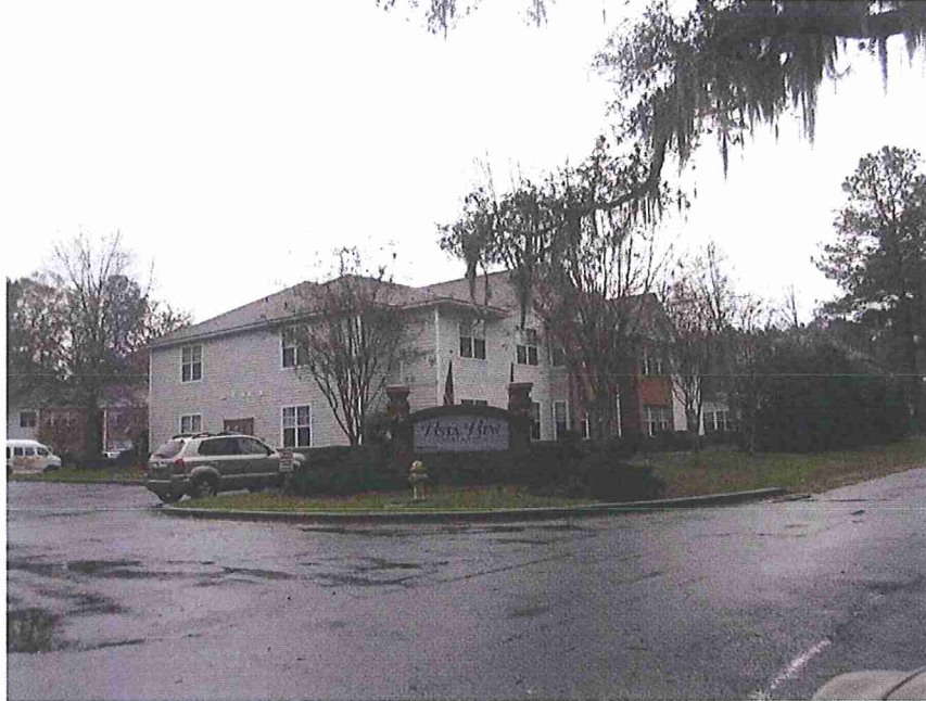
-Looking southwest at subject from site entrance
