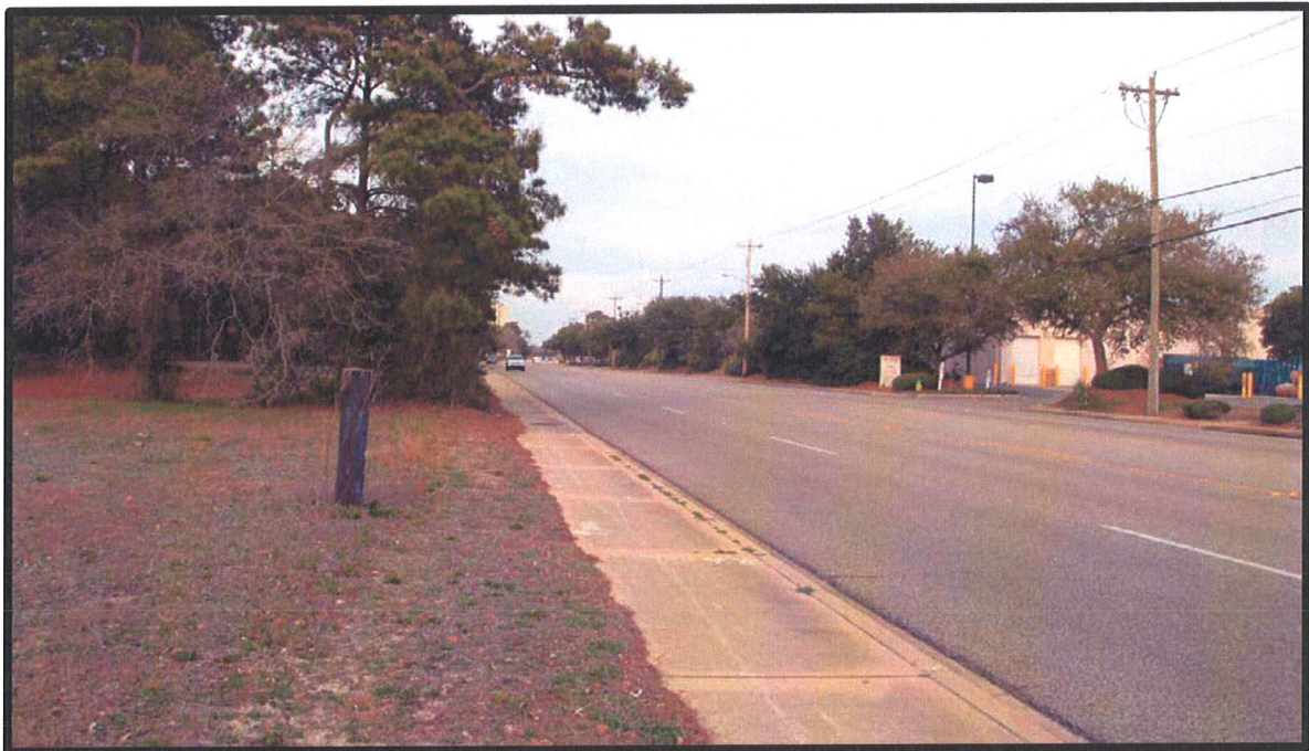
Photo 4 — On the site looking northeast on Oak Street.
