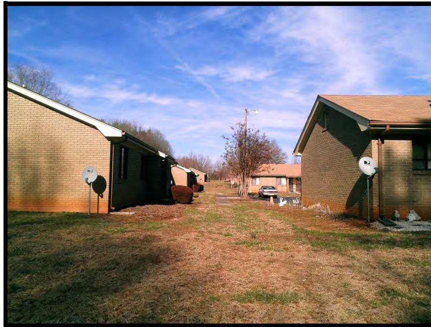
North view from site
