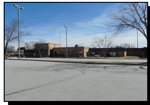
(6) West End Elementary Sch, .2 miles from site.
