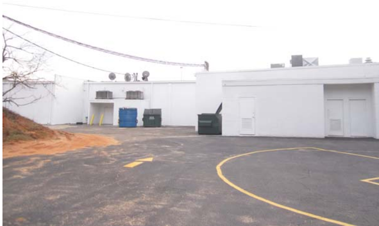
-Looking south from site boundary
