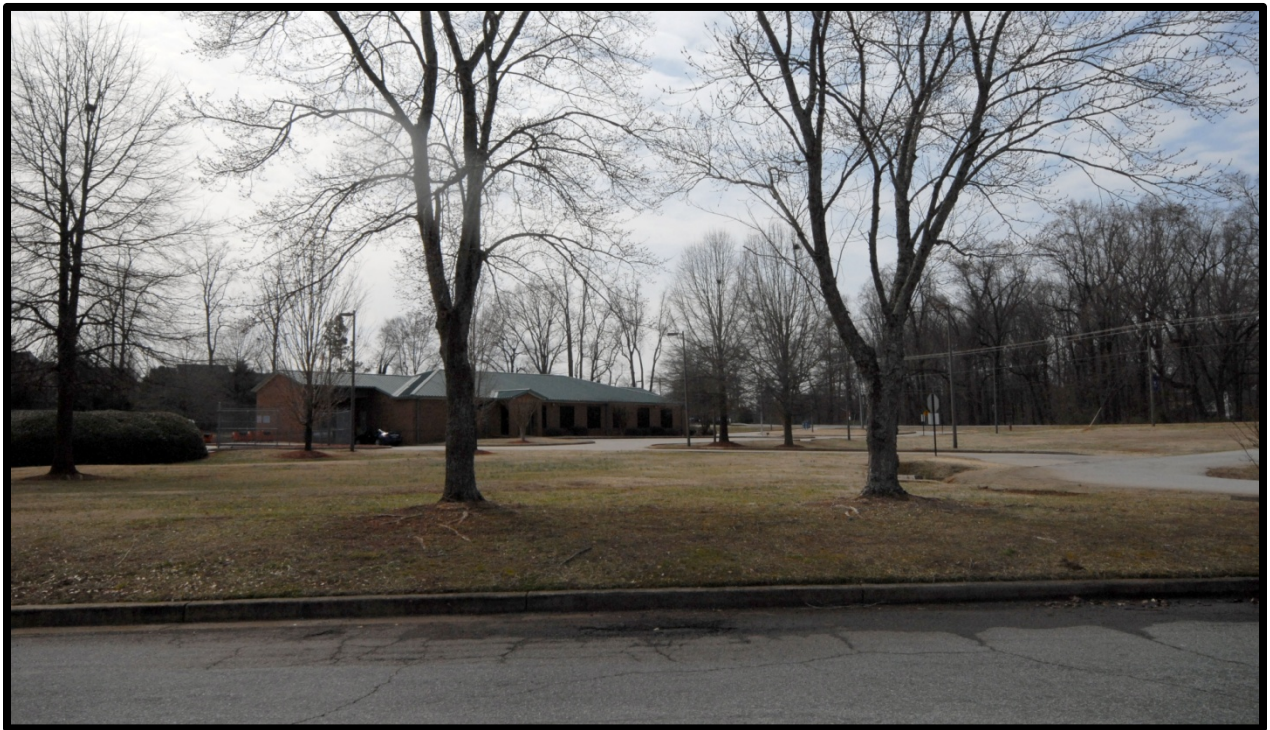
Photo 8—The U.S. Post Office adjacent to the site
