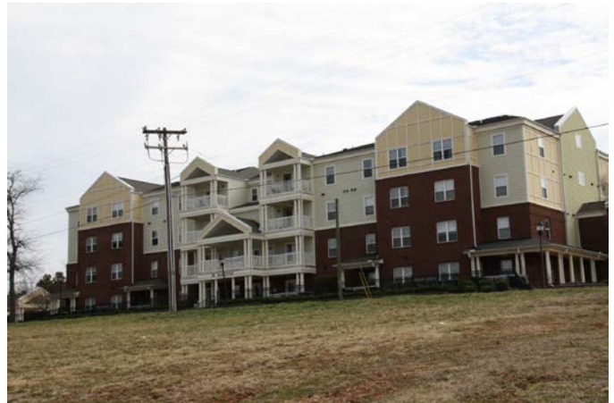
Facing east from site Charleston Place Senior Apts in distance
