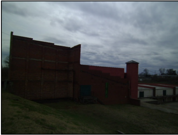
View of site and adjacent mill building, facing southwest.
