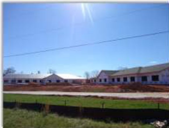
Oakview Park Assisted Living (under construction) to south.
