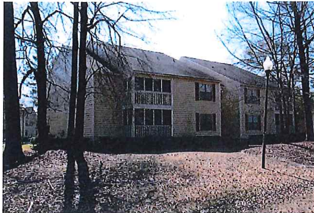
Apartments adjacent to east of site Facing east from Ladson Road
