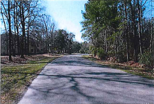
Facing south along Ladson Road Site is on right
