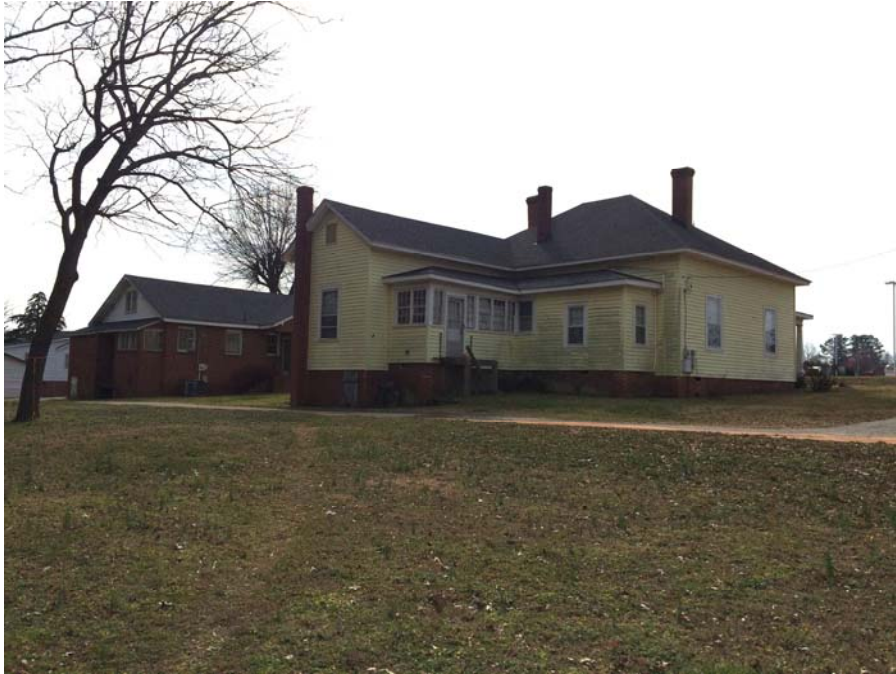
Looking south from site
