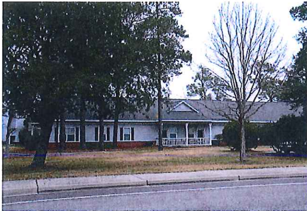
SITE – Swansgate Apartments I & II 1050 Mr. Joe White Avenue Myrtle Beach, SC Phase I – facing northeast from Mr. Joe White Avenue
