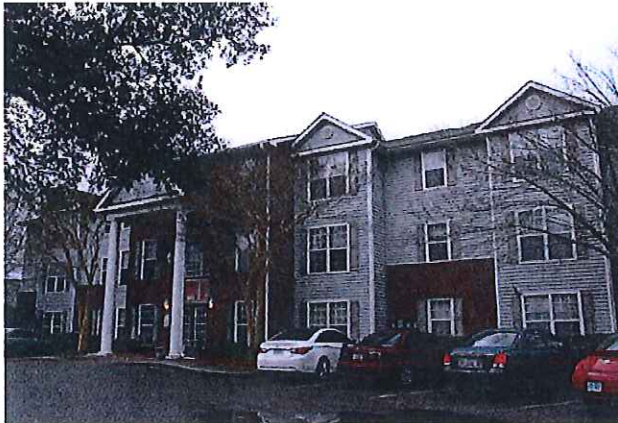
SITE – Swansgate Apartments I & II 1050 Mr. Joe White Avenue Myrtle Beach, SC Phase II – facing north from Dunbar Street
