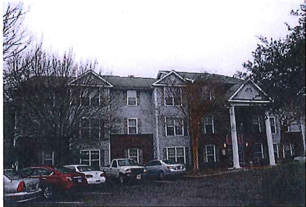
SITE – Swansgate Apartments I & II 1050 Mr. Joe White Avenue Myrtle Beach, SC Phase II – facing north from Dunbar Street
