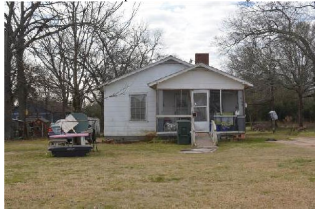
Single-family home across Laurel Street to south
