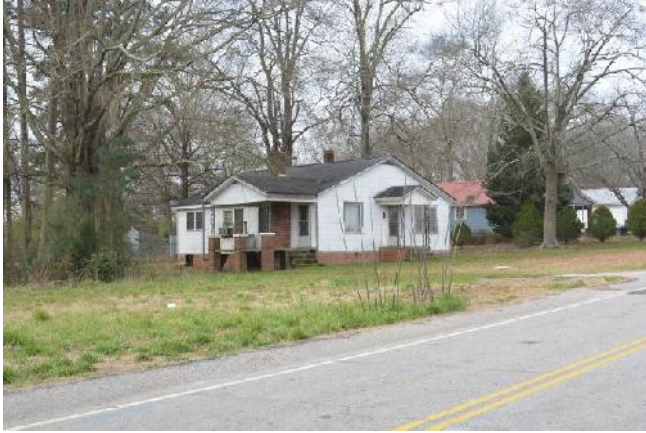
View of single-family home across from Subject site
