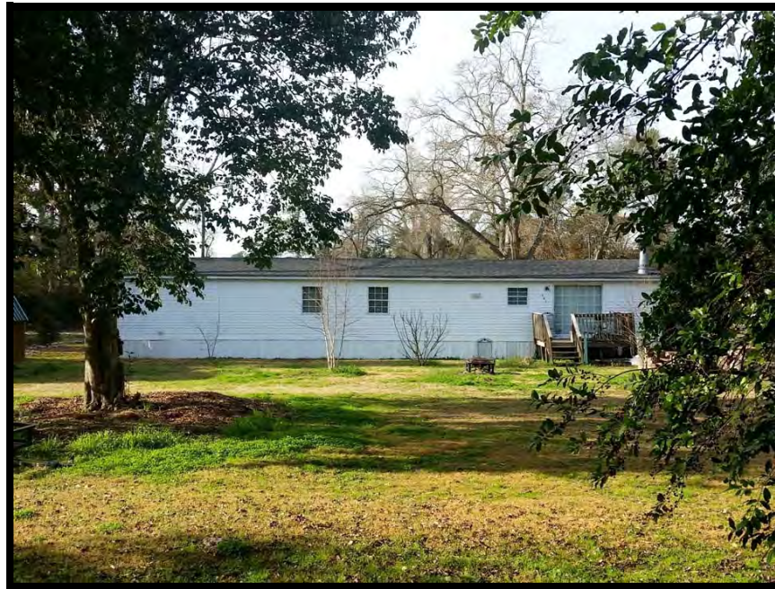
Northwest view from site
