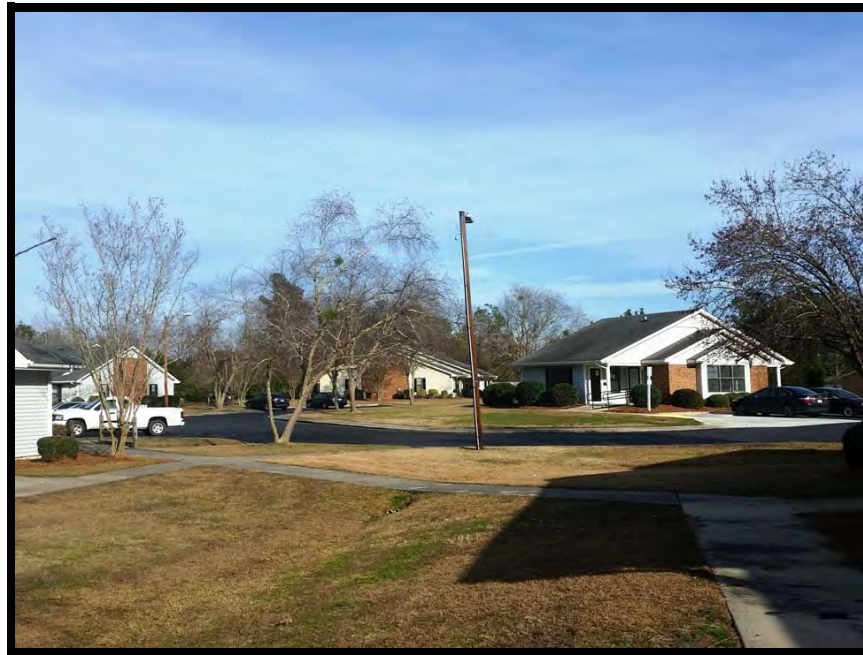
View of site from the west
