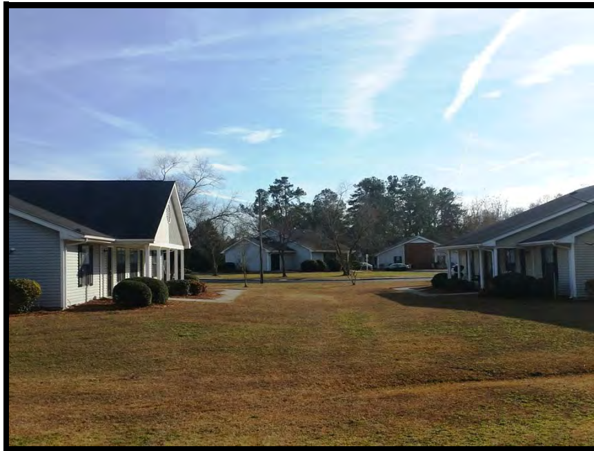
View of site from the north
