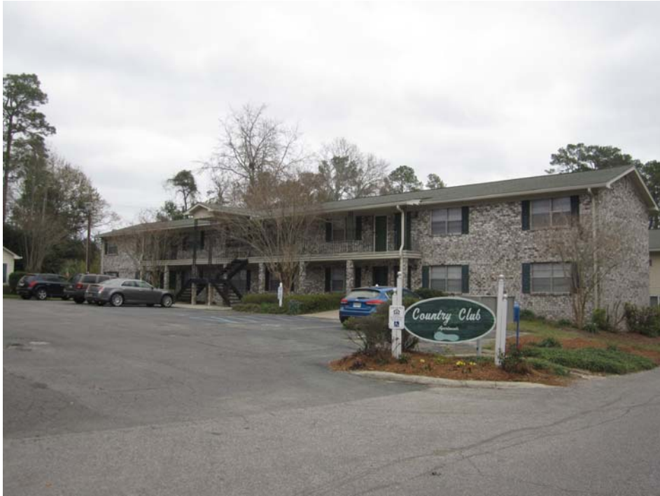
Looking northeast at subject
