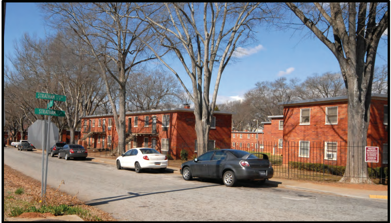
Photo 7—The subject from the corner of Stratham and Crest.
