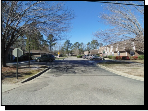
(1) Site entrance off Luden Dr, east to west.
