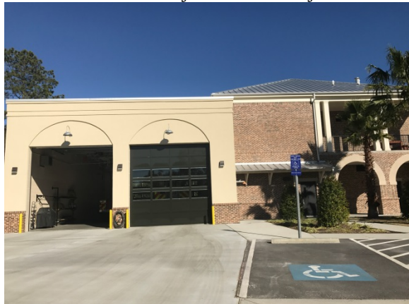
New fire station on Ribaut Road
