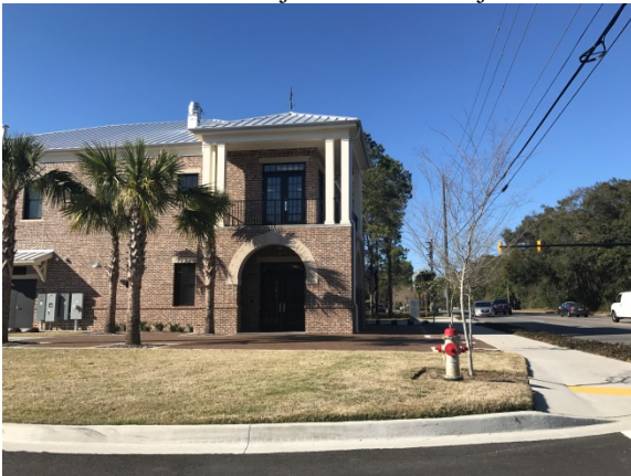
New fire station on Ribaut Road
