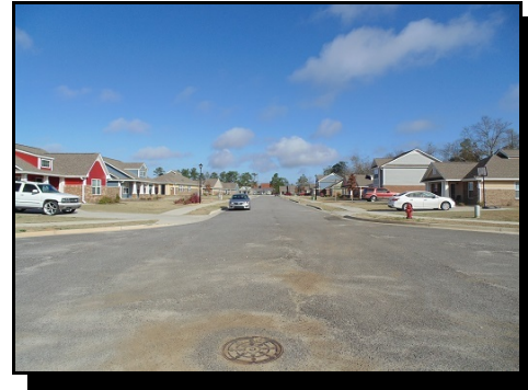
(4) From site entrance north to Dupont Landing.
