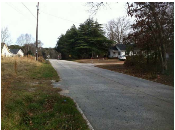
View of Suber Mill Road facing east, site on left
