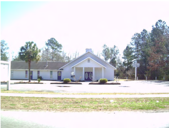
Church on Boone Hill Road, to northeast
