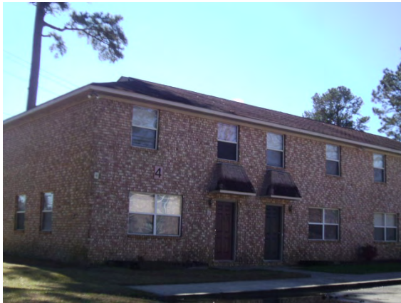
Existing townhouse building.
