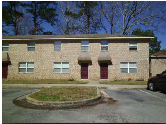
Existing townhouse building.
