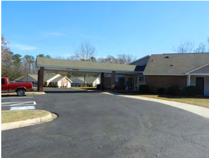
Entrance to the main building of the Subject Property.
