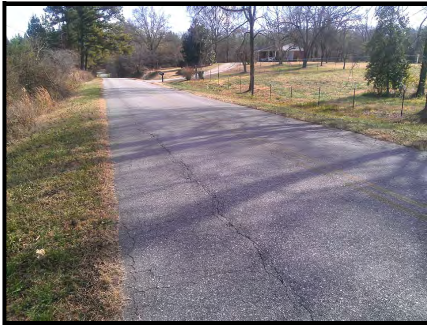
East view on Lockhart Lane
