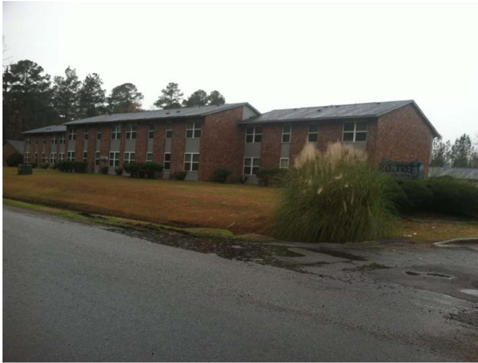
-Existing Subject Building
