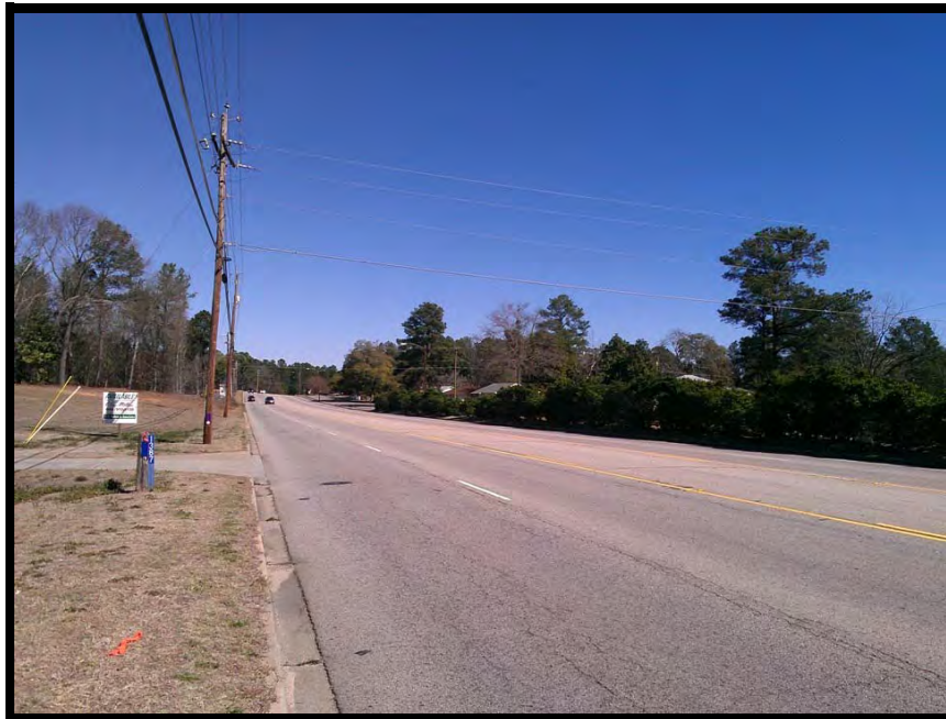
Facing north along U.S. Highway 1
