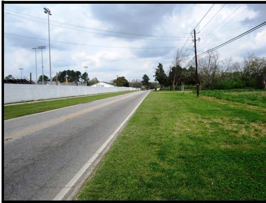
Northbound on State Route 17-39
