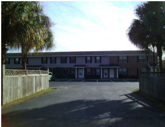
Townhomes to south along Dulsey Road.
