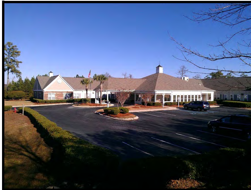
North view from site
