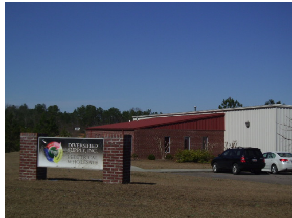
Business near subject site.
