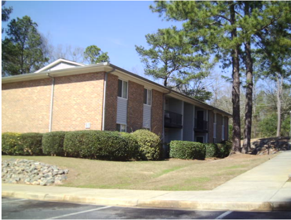
Glendale Terrace Apartments, east of site
