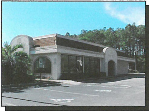
(9) Vacant Taco Bell, located south of site access point, off Frontage Road.
