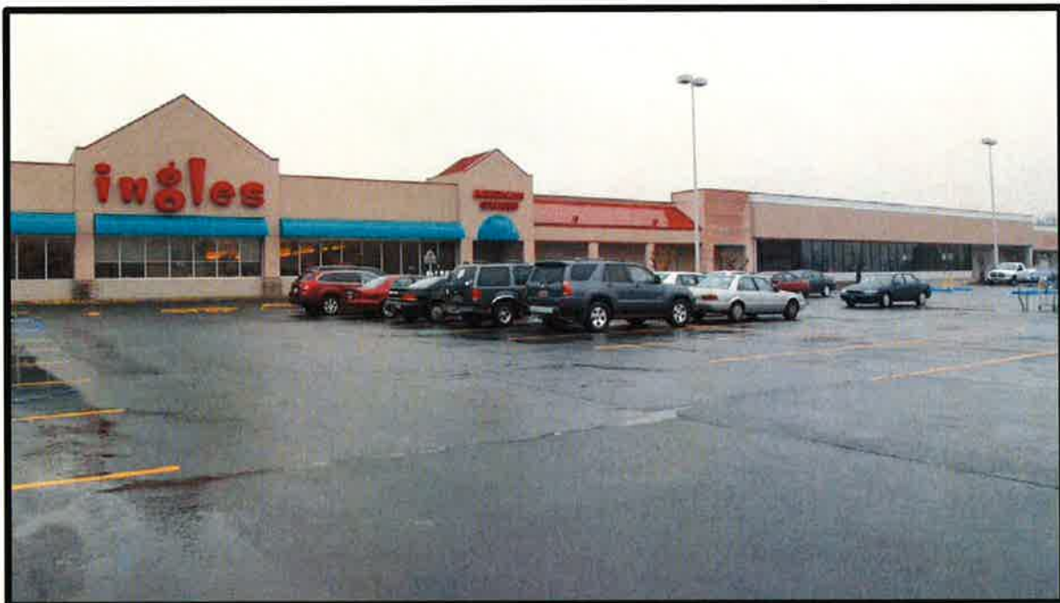
Photo 14 — The Ingles grocery across Enterprise Drive from the site.
