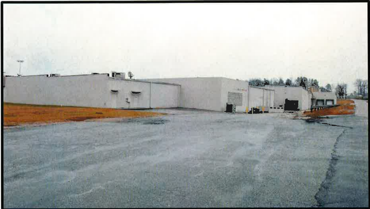
Photo 5 — The Ingles grocery store across Enterprise Drive from the site.
