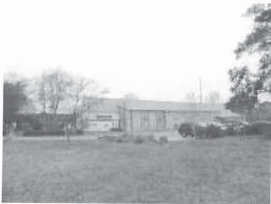
Coastalcom Building to the south of the site
