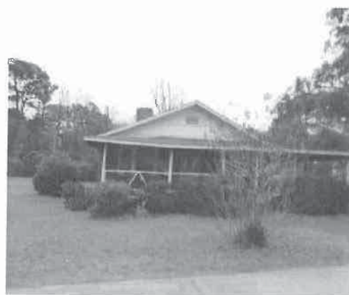
Single-family detached home west of site
