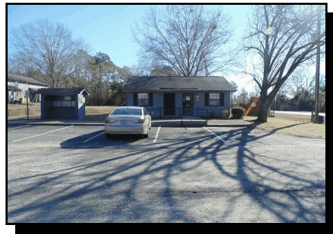
(4) Carriage Lane office.
