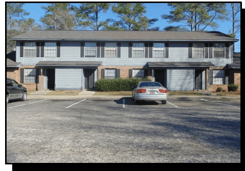
(6) Carriage Lane building.
