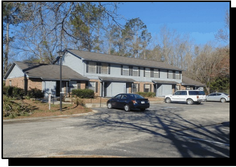
(7) Carriage Lane building.
