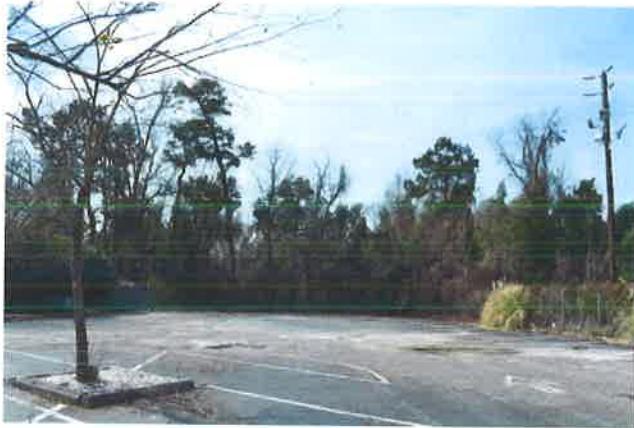
The East entrance to the Site is located behind a partially burned restaurant and next to a motel.
