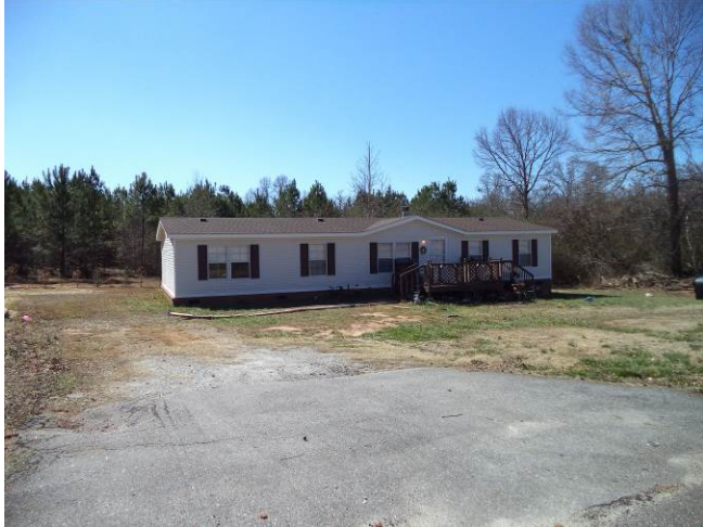
Single-family home to north
