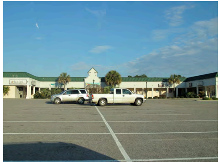
Orangeburg Mall is located across Boulevard Avenue NE from the Site.
