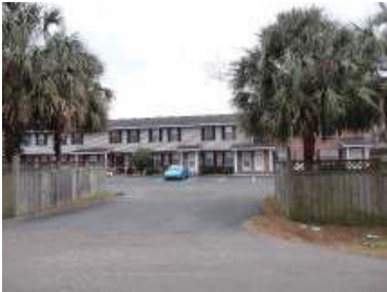
Townhomes to south along Dulsey Road.
