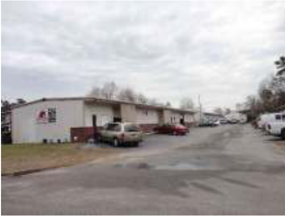
Business park to south.
