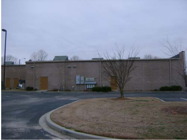
View west from Subject site of retail uses
