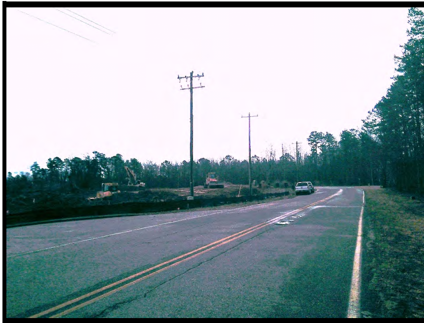
South view along Willis Road
