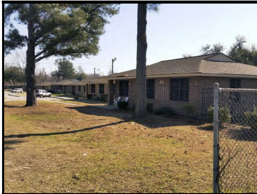
View East of Site
