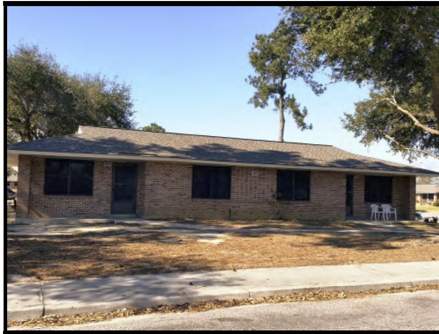
Typical building adjacent site
