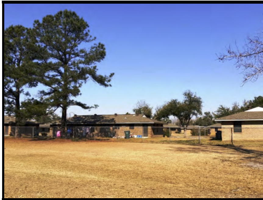
Northeast view from site
