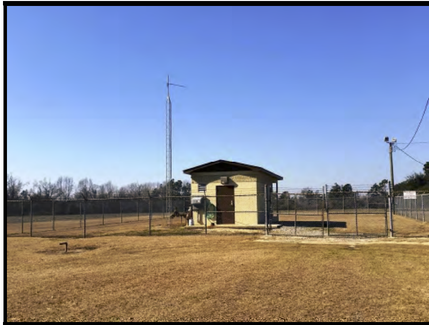
Well adjacent site
