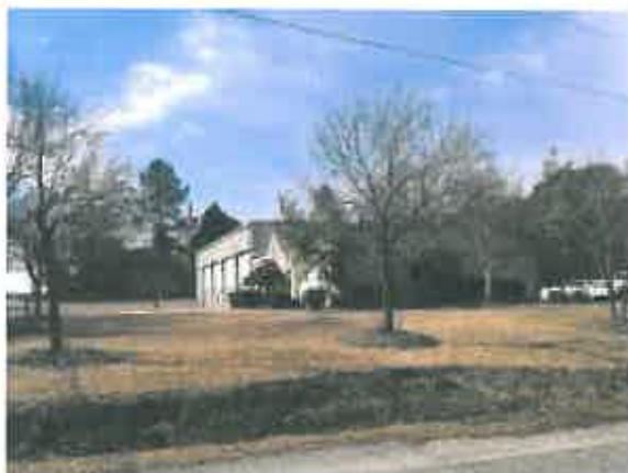
Columbia Fire Station 26 just north of the site
