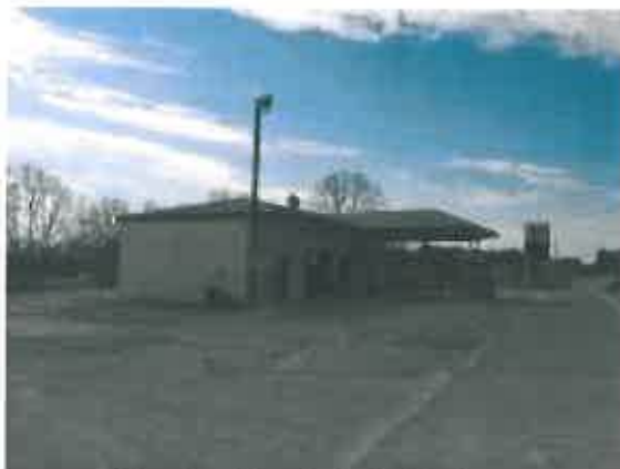
BP service station bordering the site to the east
