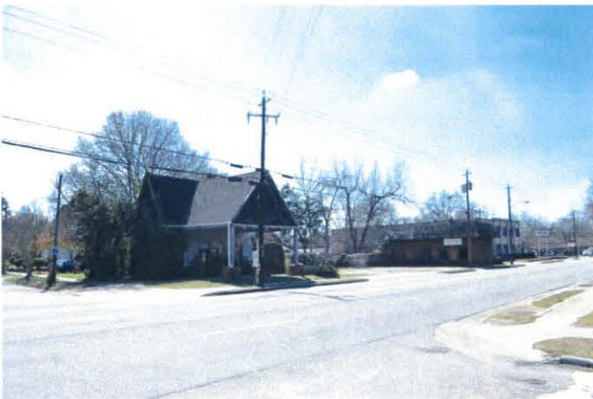
Two old abandoned buildings are located to the South of the Site across West Liberty Street.
