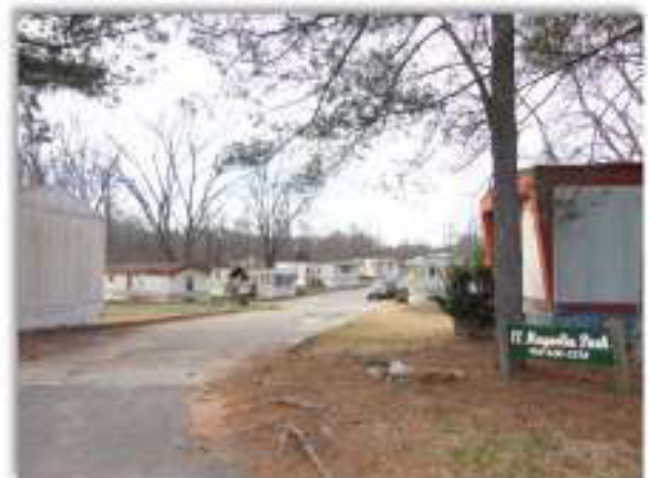
Mobile-home park to the north.
