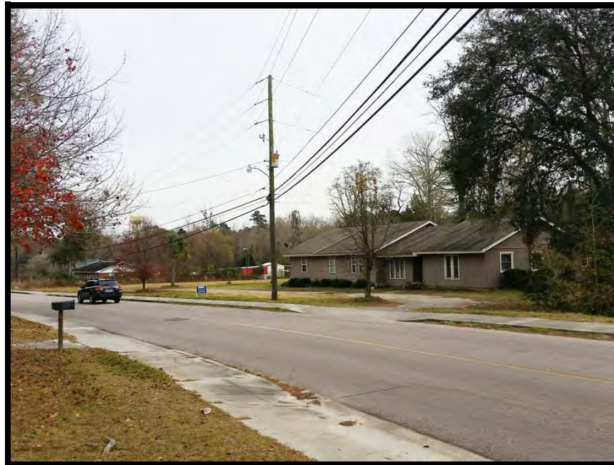
Southeast view from site
