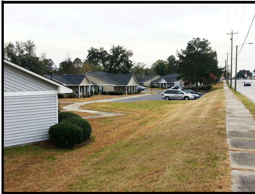
View of site from the north
