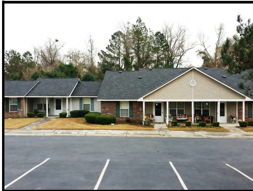
View of site from the west
