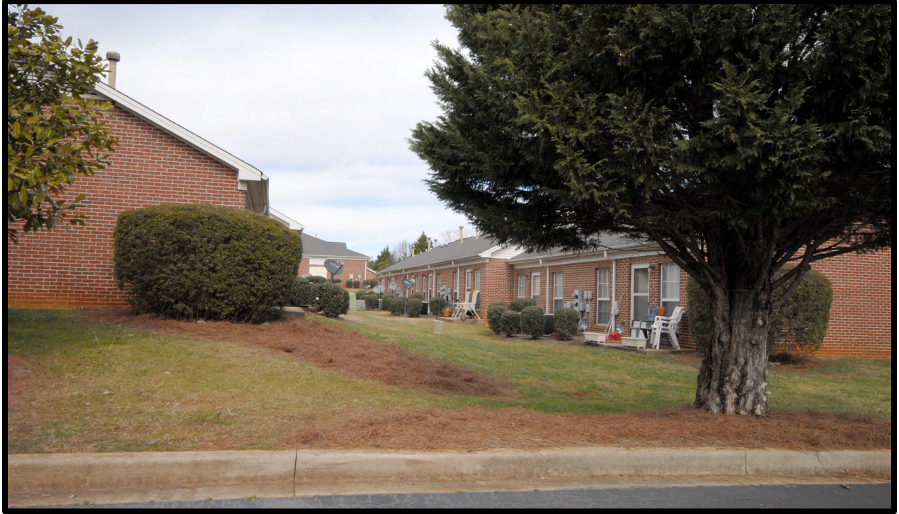
Photo 3—Area between the backs of the buildings.
